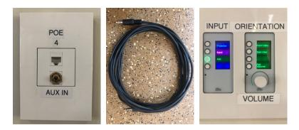
To control the sound level, first be sure the output level of your source device is turned up to at least 75%, then be sure the **INPUT** control is switched to **Aux** (bottom button, green background), and adjust the volume knob as desired.
